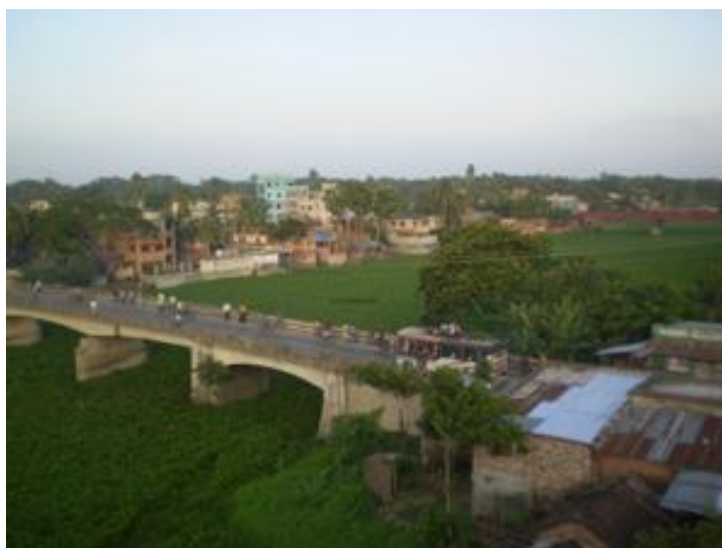
Photograph 10.1: Jhikorgachha Bridge over Kobadak
