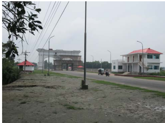
Photograph 10.4: Benapole Gate under construction
