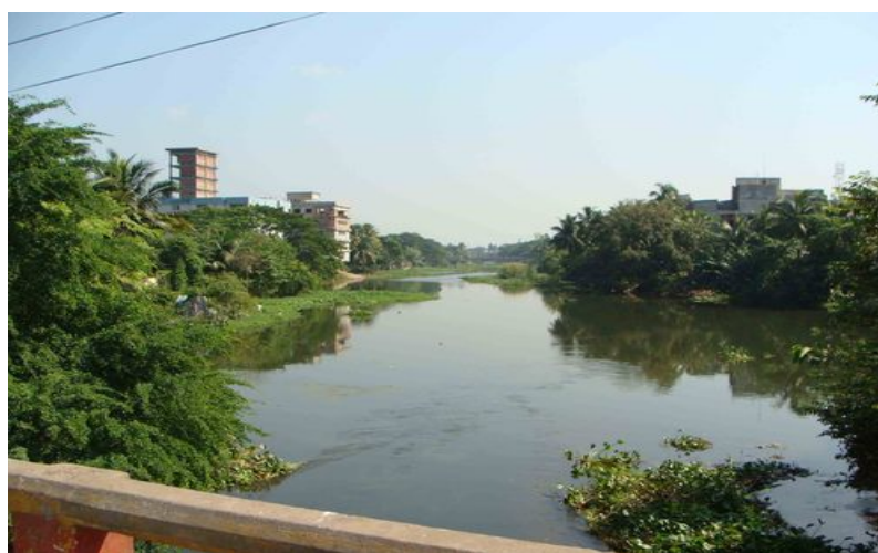
Photograph 10.2: Daratana Bridge over the Mukteswari River at Jessore Town and encroachments from both ends of the river
