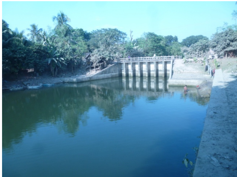
Photograph 3.3: The newly constructed regulator (BWDB design) close to water structure (British design) at the mouth of Kata Khal joining the Kobadak River at Jhikargacha.
